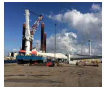
Windlift 1 for Bard Offshore Wagenborg, Julianahaven
