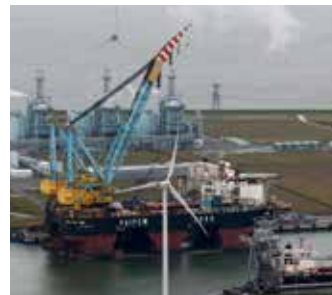
Saipem 7000 (maintenance) Wilhelminahaven
