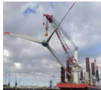
MPI Adventure for Trianel Borkum Buss Terminal Eemshaven, Julianahaven
