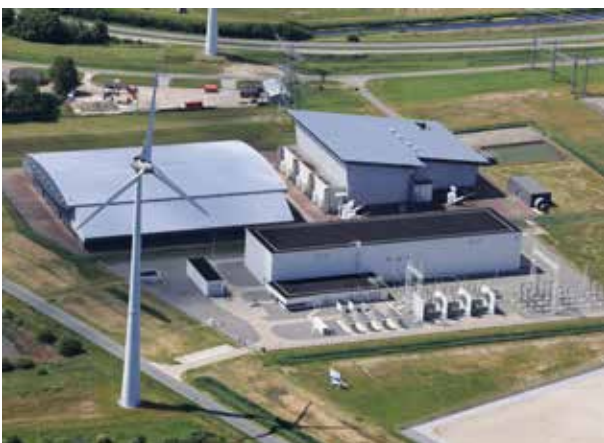
Converter station TenneT | NorNed (above) - undersea high voltage cable between Eemshaven (NL) and Feda (N) and TenneT | COBRA (under) - cable between Eemshaven (NL) and Endrup (DK).
