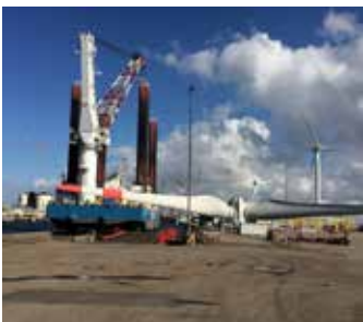
Windlift 1 for Bard Offshore Wagenborg, Julianahaven
