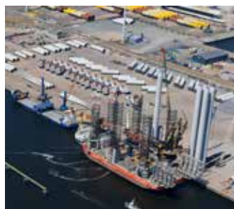
Wind Osprey for Hollandse Kust Noord Buss Terminal Eemshaven, Julianahaven
