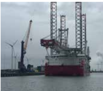
Seajacks Scylla for Veja Mate Buss Terminal Eemshaven, Julianahaven
